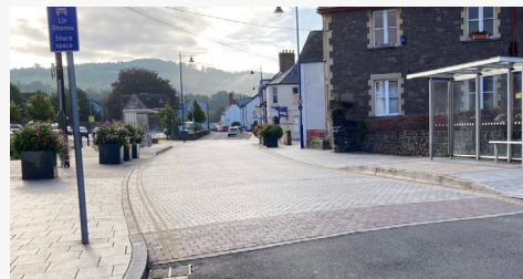
↑ Example of a short length of raised shared surface on a 20mph high street with road edge markings (Abergavenny).
